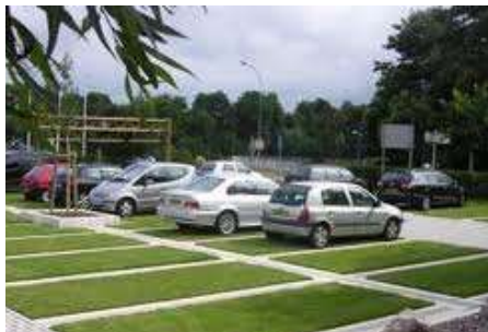
Parking perméable – Source : www.ecovegetal.fr
